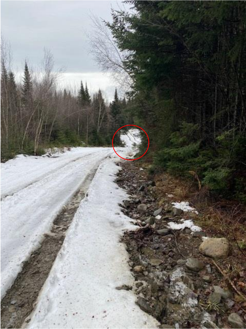
Hudson Road Left Ditch (culvert location in red circle)
